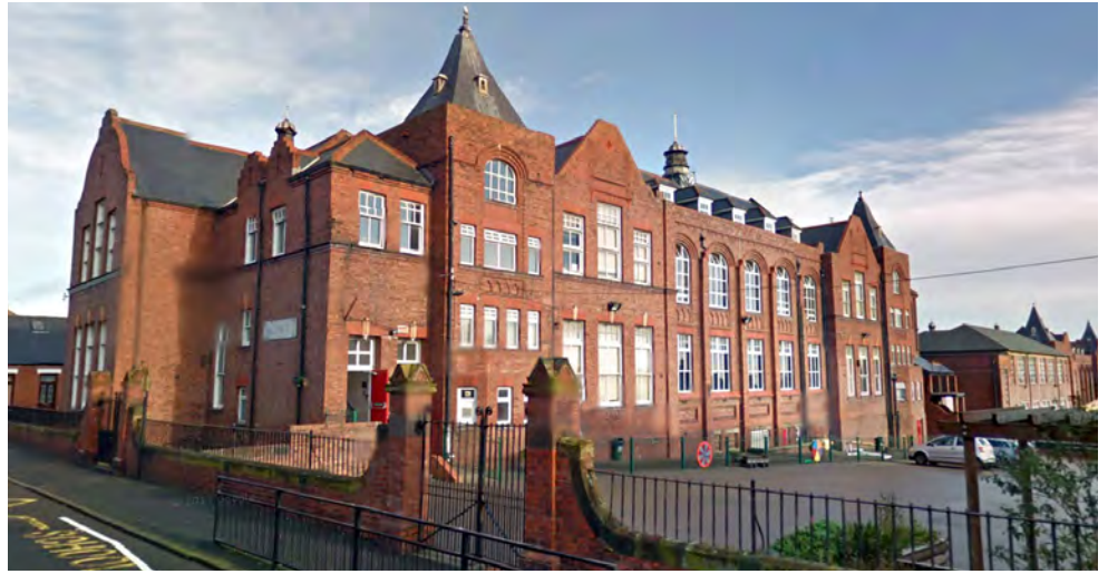
In July 1902, J B Wilkinson carried out the plumbing installation to the new schools that were opened at Wycliffe Road, High Barnes, Sunderland.
